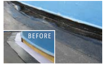
Double-bottom tank sealed with PolySeam prevents water from going under the tank, no corrosion.
