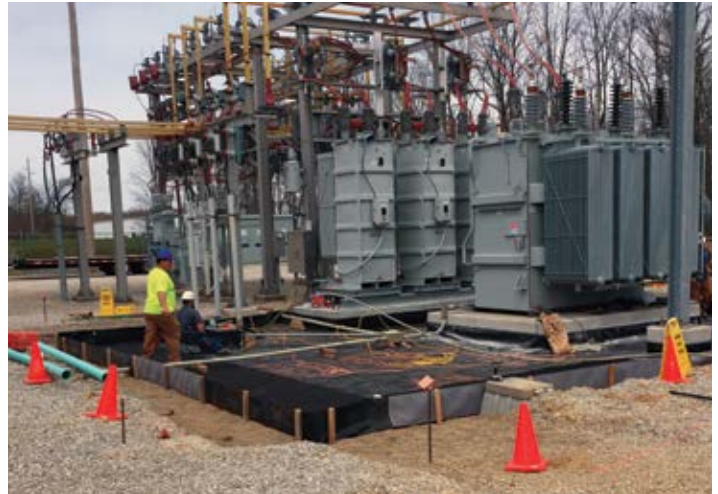
Geomembrane Liner with Barrier Boom oil containment system during installation.
