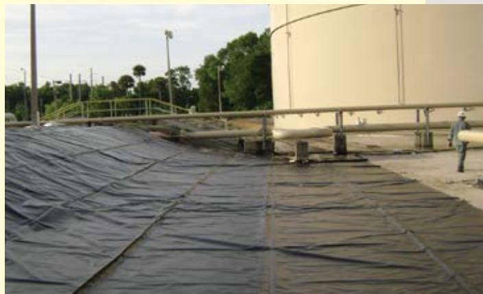
Completed installation providing reliable, safe secondary containment for 3-million gallons of diesel fuel.
