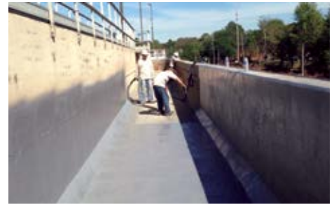
Spray-on technology coats smoothly to repair cracks and leaks—tack-free in seconds
