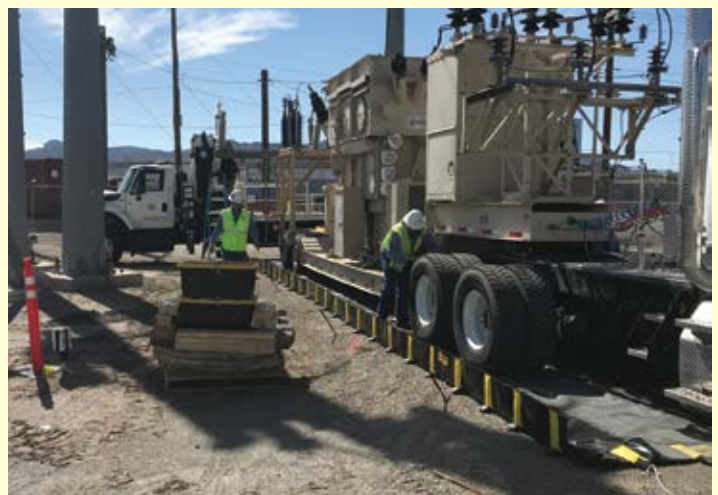
Rigid-Lock QuickBerm and HFF Oil Stop Valve provides leakproof protection and captures hydrocarbons for mobile transformer.
