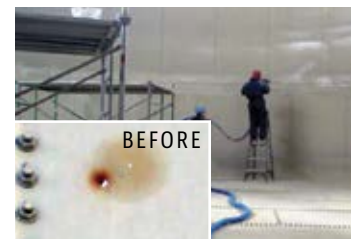
Holes in tank were repaired using our structural coating system
