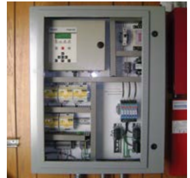
Control panel monitors up to 128 sensor circuits simultaneously
